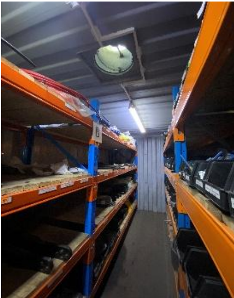
Photo 19 This container stores illumination level comply with 75 Lux requirement
