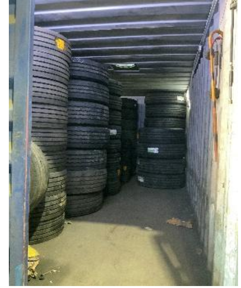
Photo 22 Illumination of the tyre container storage unit does not comply
