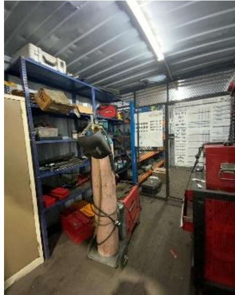
Photo 17 Illumination levels in this Container workshop store complies with 100 lux requirements
