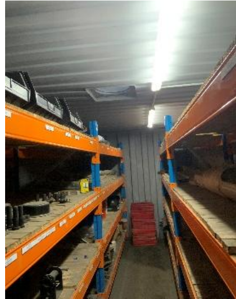
Photo 18 Illumination in this storage container in the Workshop complies with 100 Lux requirement for component storage
